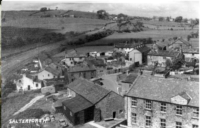
The view from the old mill chimney. The large building in the foreground is Broadstones Farm. This was demolished when Silentnight created their car park
