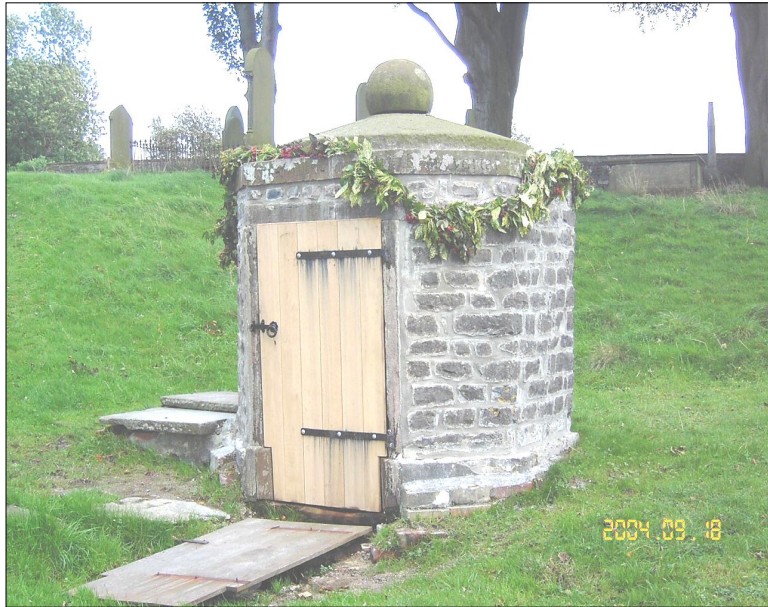
The Refurbished Well
