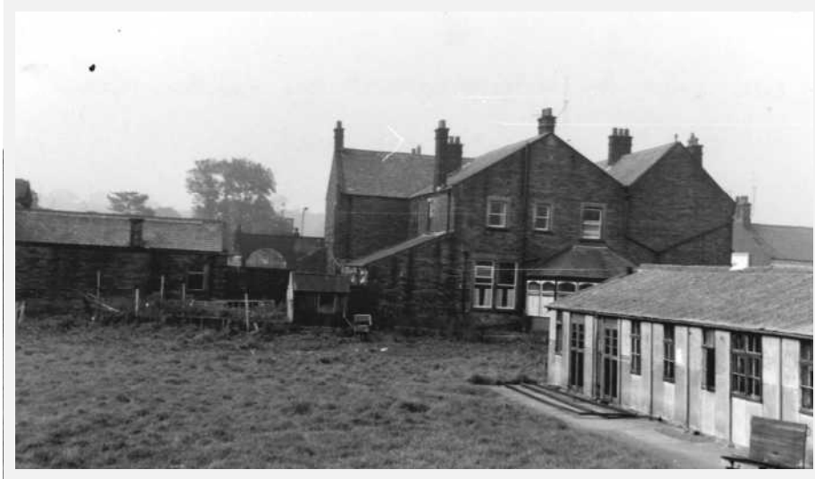
Rear of Station Hotel with Nursery
