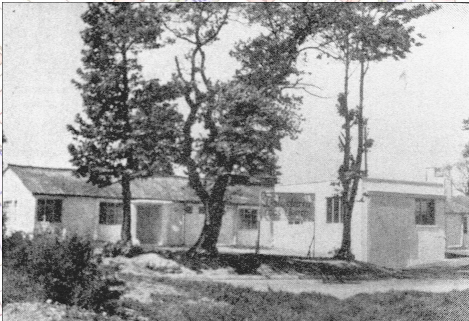
The Section of the Building used for the egg packing station with loading facility extension to the front
