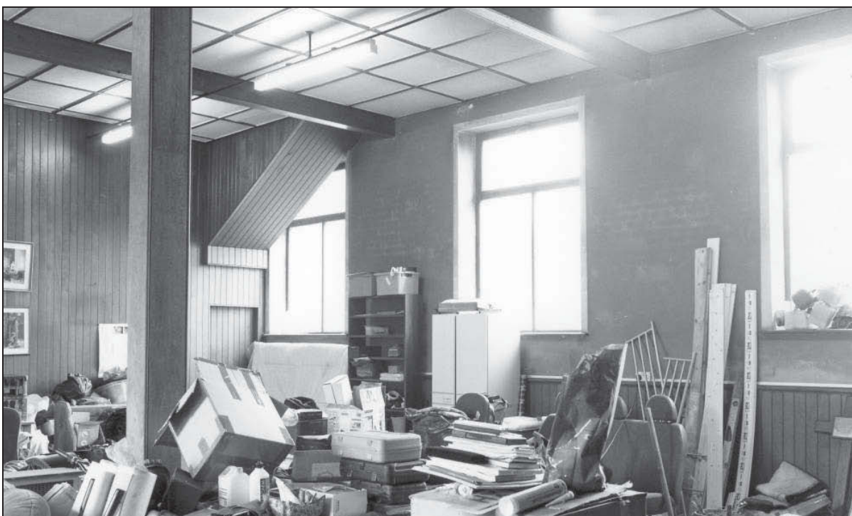
Photo 60: The school room, from the east
