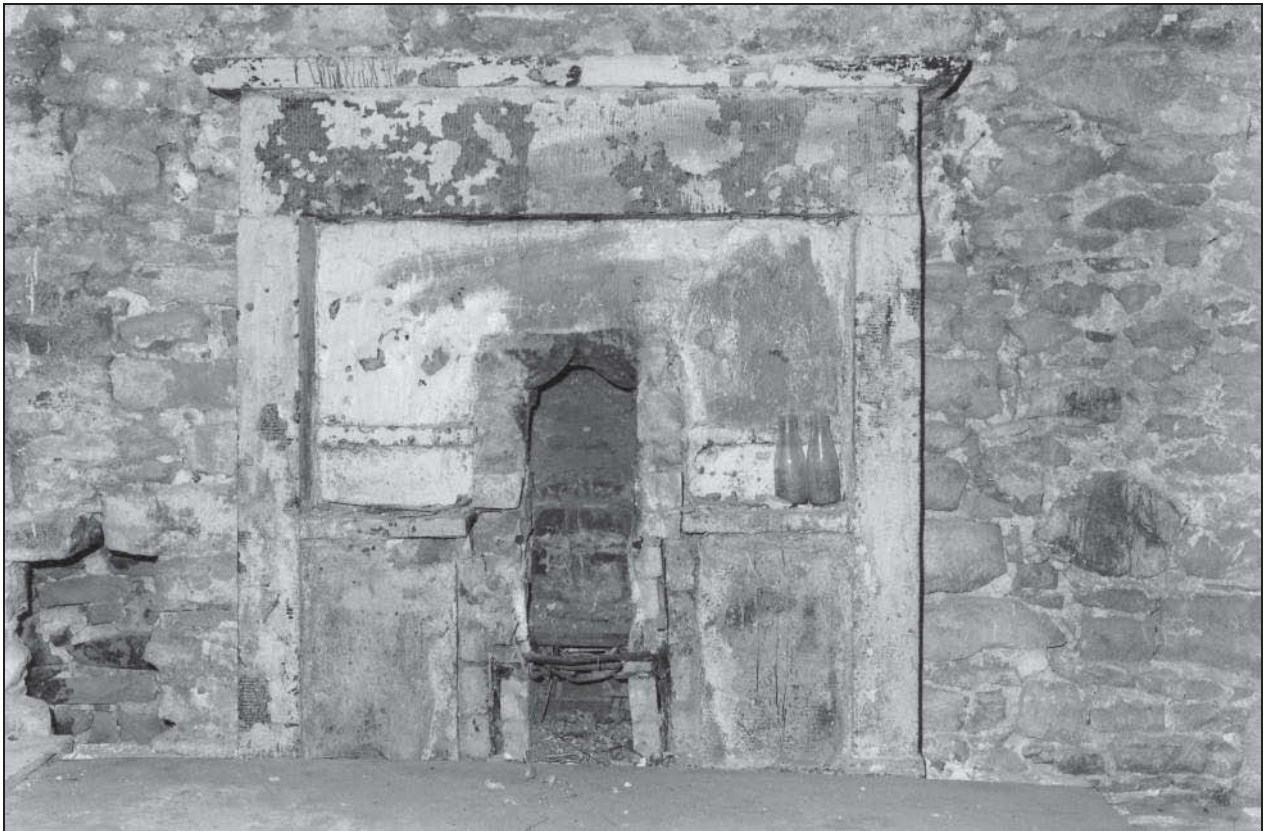
Photo 88: The outbuilding: first floor fireplace
