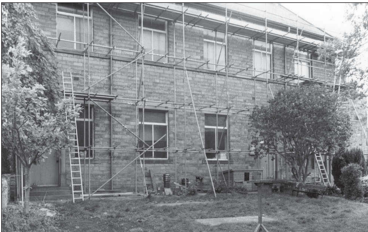
Photo 3: South-east elevation of the church
