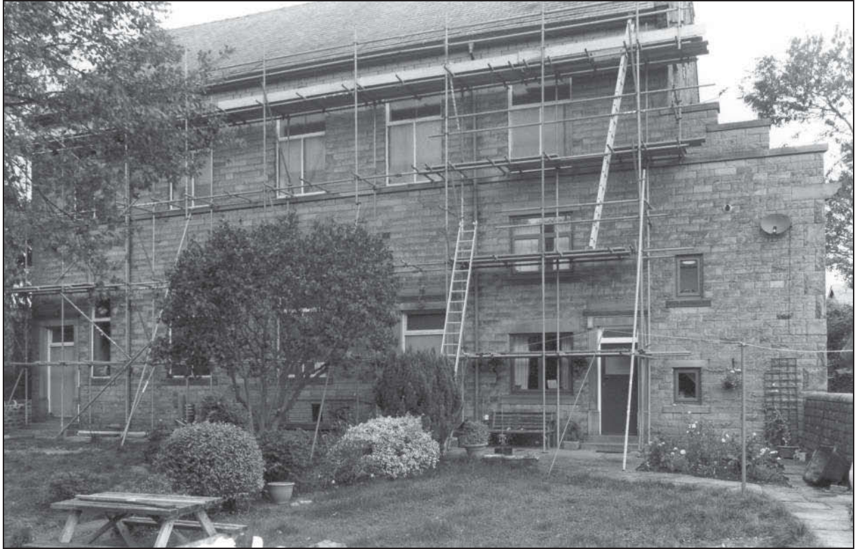
Photo 4: South-east elevation of the church, and caretaker's house to right
