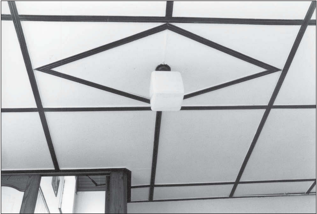
Photo 31: Main entrance lobby to church: detail of ceiling
