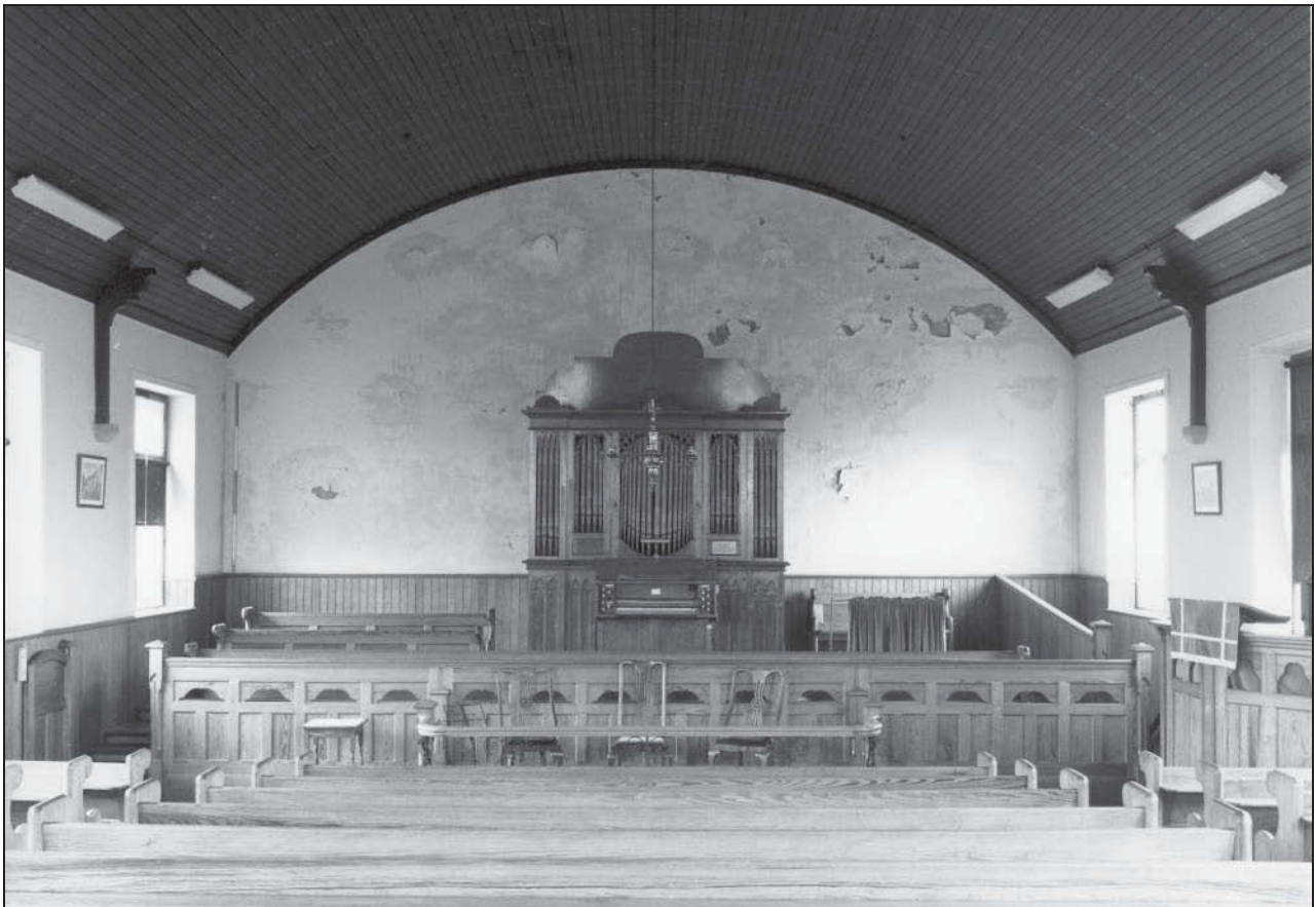
Photo 33: The chapel, from the north-east end
