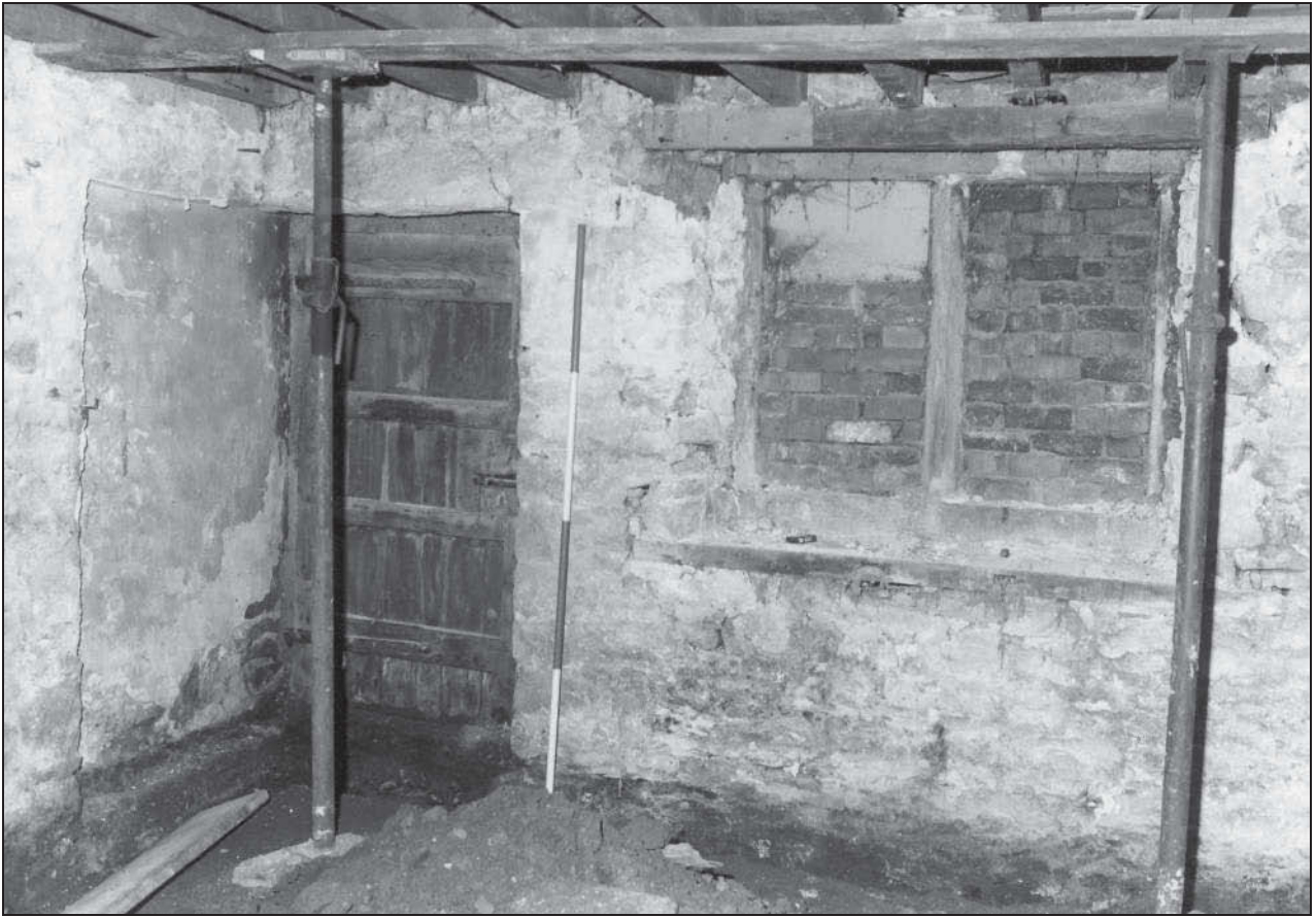
Photo 81: The outbuilding: ground floor, from the north-west
