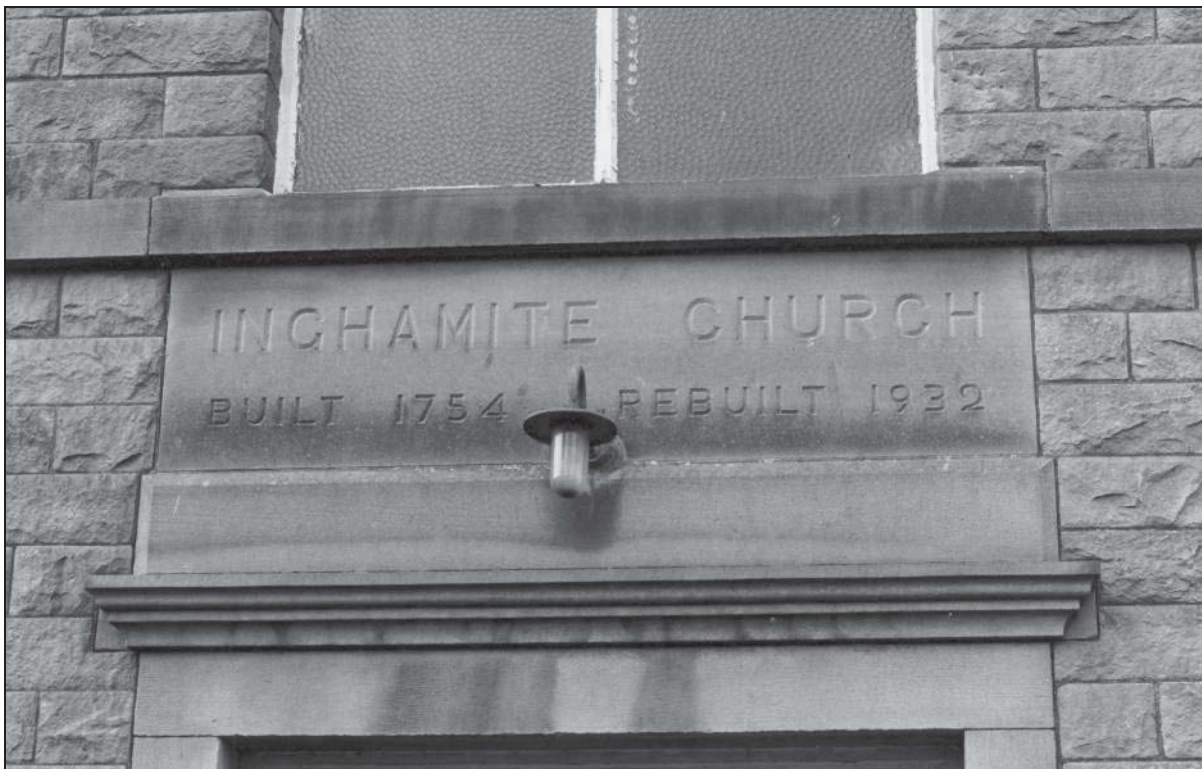
Photo 18: North-west elevation of the church: inscription over main entrance
