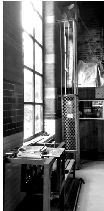
Picture 2 The clock base structure and tower for winding weight being installed at Bancroft Mill
