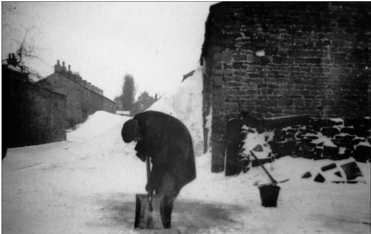
Snow Drifts at the junction of New Road and Green End Road
