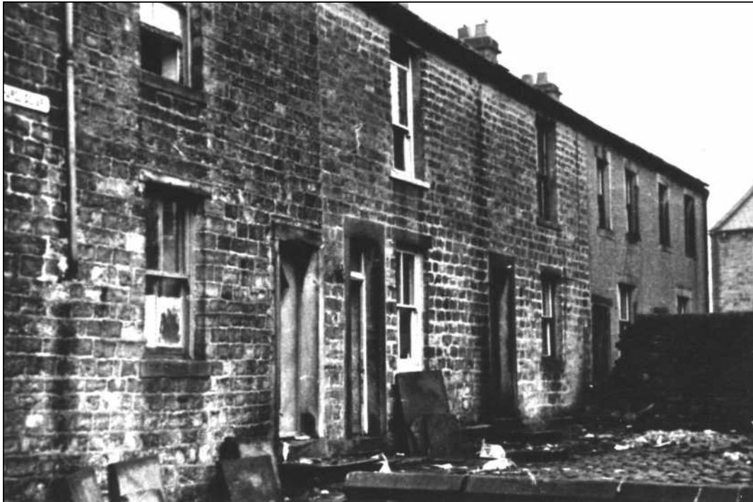
The photograph above shows the old Chapel and adjoining buildings before demolition. The house on the left was the Minister's residence (adjacent to Red Lion Street). The next two were the original Chapel and past the wall are the two houses of Earlham Street. Careful observation shows the position of the gable end walls of the original Chapel buildings.
