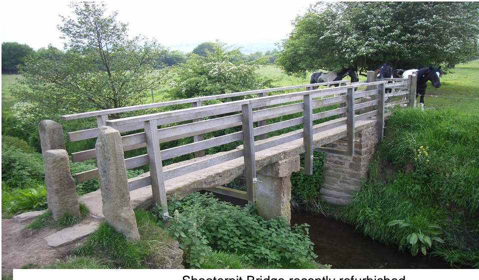
Shooterpit Bridge recently refurbished
