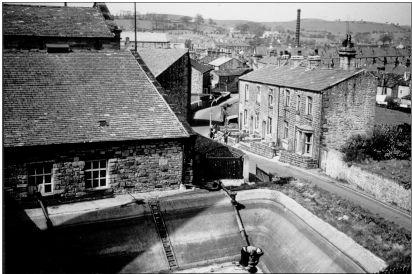
The front of Spring Mill with the lodge for storage of water for the boiler Photo by the late Dave Sedman
